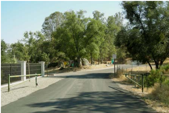
Two steel pipes on hinged posts form the gates.
