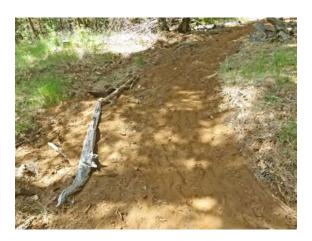
We then laid brush and small logs along the outside turns of the new trail so that horses are visually guided. Side-drainage swales are thereby concealed, and the horse's eyes focus on the proper trail route. In future years, grass will grow along the outside edge of the trail and the limbs will rot away.
