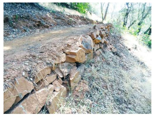
These are Copper Hill Volcanics of the Jurassic Period. These blue-gray metavolcanic rocks have been sheared along the nearby Bear Mountains Fault Zone ( $\approx$  one mile northeast) so that foliation planes are well-developed with a strike azimuth of N±30°W, and near-vertical dip ±80°SW. During 2012 trail construction, these flat boulders were cleverly used by Donald R. Hays, licensed professional trail builder, to strengthen the outside shoulder of Creekside Trail.
