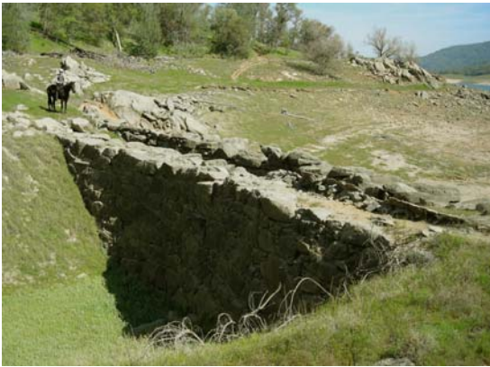
Stone viaduct along the North Fork Ditch.
