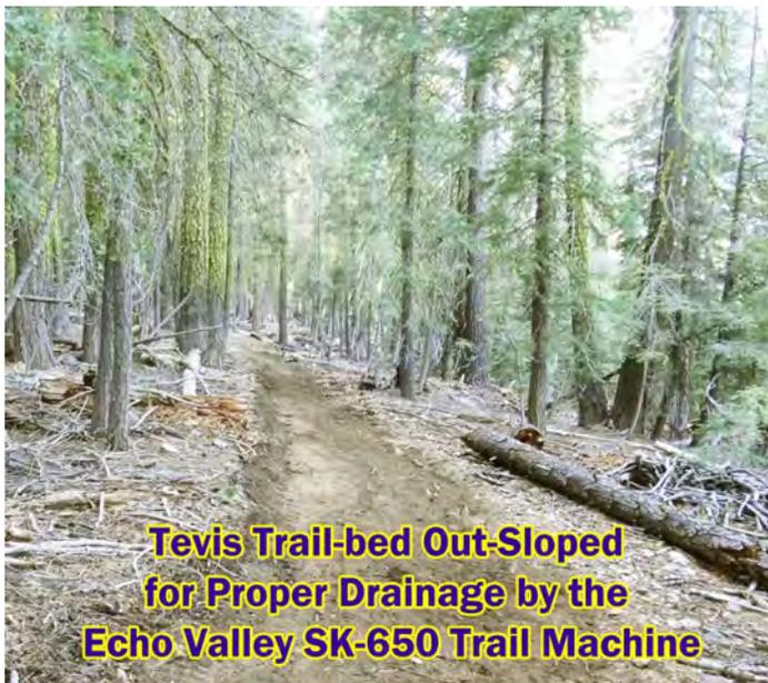
**Tevis Trail-bed Out-Sloped for Proper Drainage by the Echo Valley SK-650 Trail Machine**
