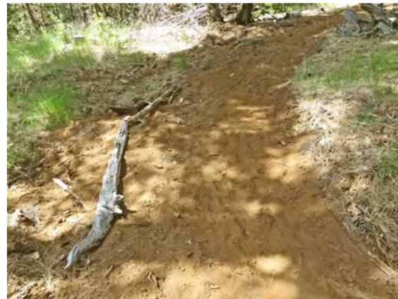
We then laid brush and small logs along the outside turns of the new trail so that horses are visually guided. Side-drainage swales are thereby concealed, and the horse's eyes focus on the proper trail route. In future years, grass will grow along the outside edge of the trail and the limbs will rot away.
